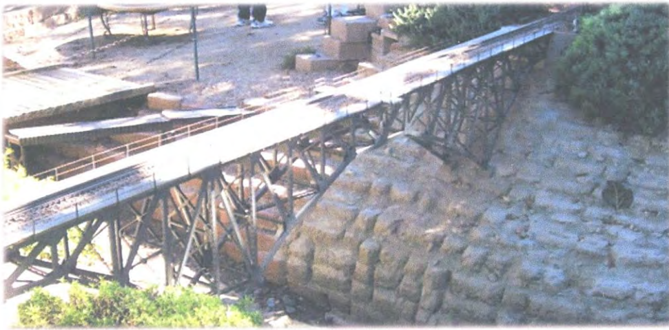
A better view of the bridge itself.
